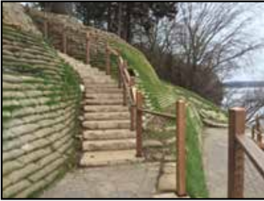
Stone steps and hand rail ascending the slope.
