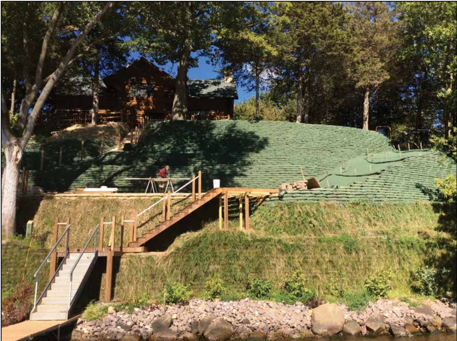
Completed Envirolok progress from the fall of 2015.
